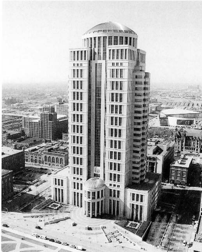
Thomas F. Eagleton Federal Courthouse, St. Louis, Missouri, 2000. Architects: Hellmuth, Obata + Kassabaum, Inc. Figure 39.
