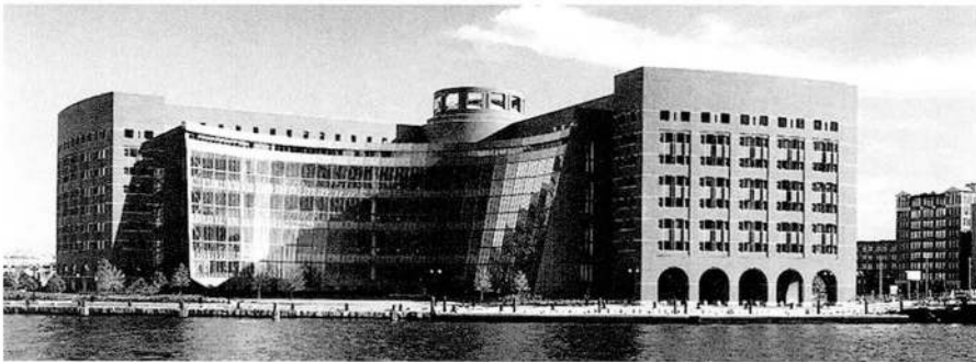
John Joseph Moakley United States Courthouse, Boston, Massachusetts. Architect Harry Cobb, 1998. Figure 29.
