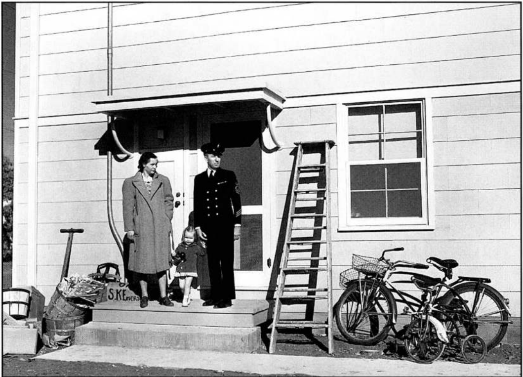
Fear that rents would soar in places where defense workers sought housing prompted passage of the Emergency Price Control Act's provision that rents be controlled in areas near military installations and war industries. Above, a defense worker and his family posed outside their home near a naval base in Connecticut.
