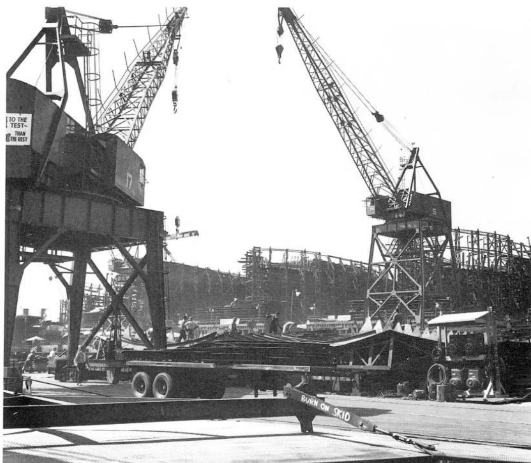
The construction of the Booker T. Washington , the first liberty ship named for an African-American. Booker T. Washington was built at the California Shipyards Corporation in Los Angeles, although liberty ships were being built around the country.
