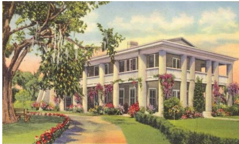
Fleeing arrest and prosecution for war crimes following the collapse of the Confederacy, Benjamin took refuge in the Gamble Mansion (above) with a famous Confederate blockade runner, Capt. Archibald McNeill. The mansion still stands near Bradenton, FL.
