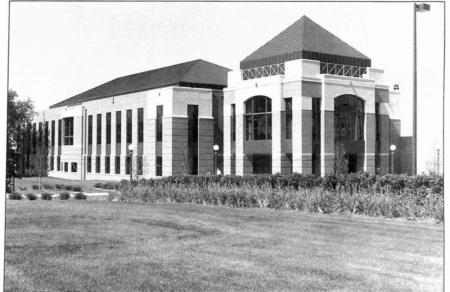
The Warren E. Burger Library at William Mitchell College of Law was designed by Winsor/Faricy Architects, Inc. of St. Paul. Groundbreaking for construction of the building took place in spring 1989.
