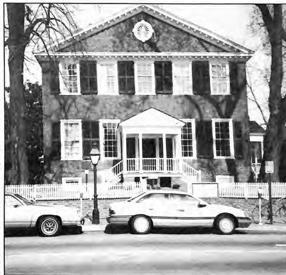
The John Marshall house in Richmond, Virginia
