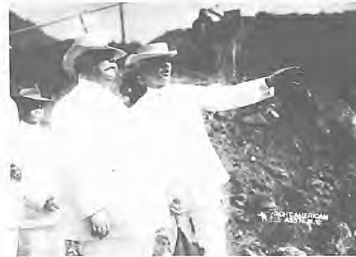
Taft supervises construction of the Panama Canal during his tenure as Secretary of War.
