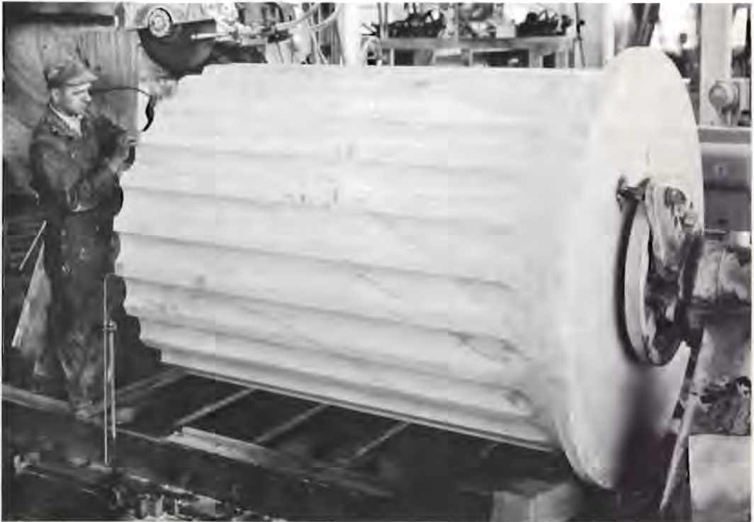
A workman is all but dwarfed by the section of column on which the finishing touches are being applied.
